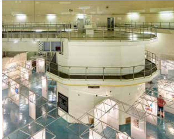
Since 1996, the FR2 has been in the state of safe enclosure. The reactor hall accommodates a nuclear technology exhibition.
