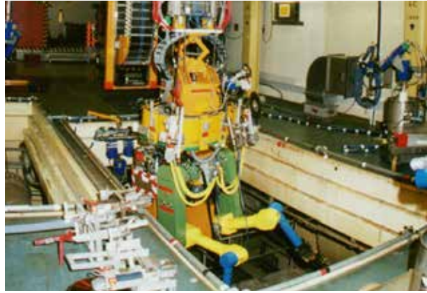
Remote dismantling of process installations.
