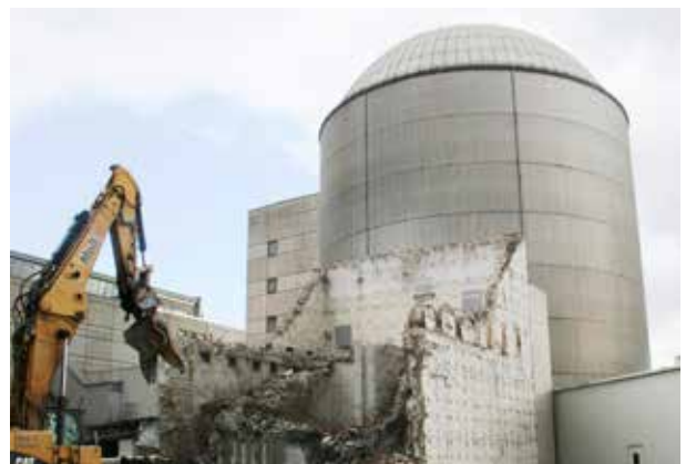
Direct dismantling of the Multi-Purpose Research Reactor.
