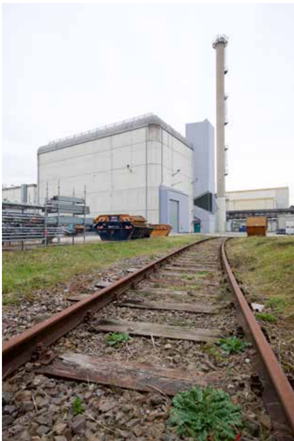
Transportation of glass canisters in Castor casks is history. Now, complete dismantling of the VEK has to be managed.
