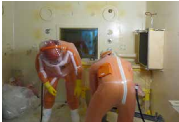
Specialized staff dismantles cell internals.
