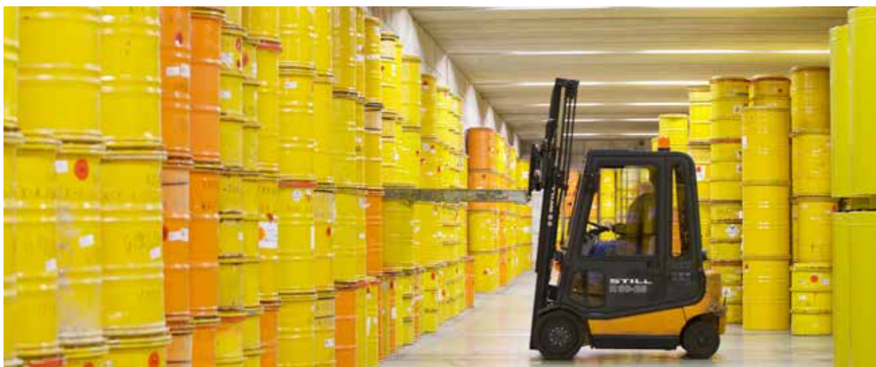
Stored waste packages are controlled constantly.
