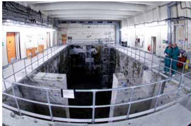
Emptied, pitted, and decontaminated: The fuel element storage pool today.
