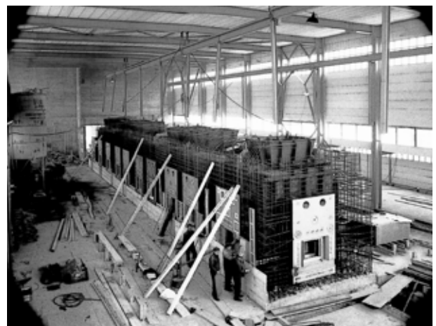
The large concrete cells were built in 1964 and operated until the mid-1990s.
